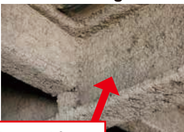
Steel frame fireproof coating
